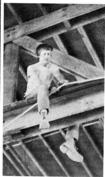
Scott Thompson assembles conduit 20 feet up in the car shop rafters.
