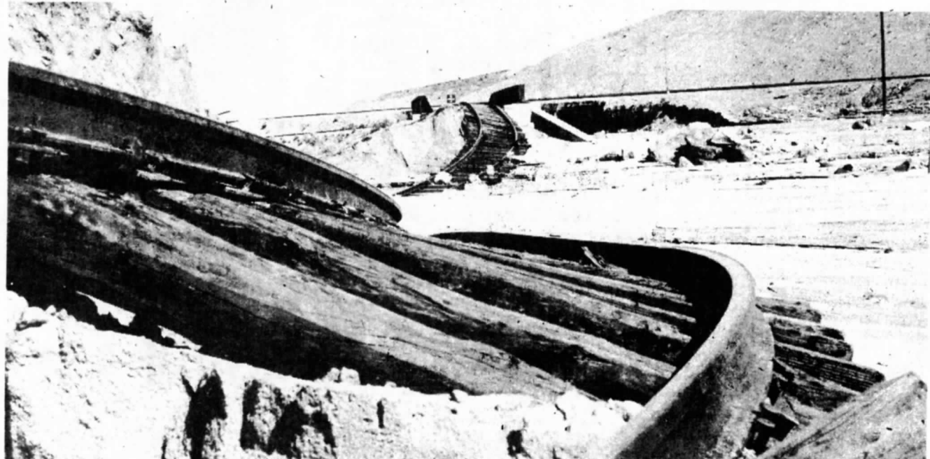
Twisted track and warped ties on the roadbed of the San Diego and Arizona Eastern Railway mark the path of tropical storm Kathleen in September.
