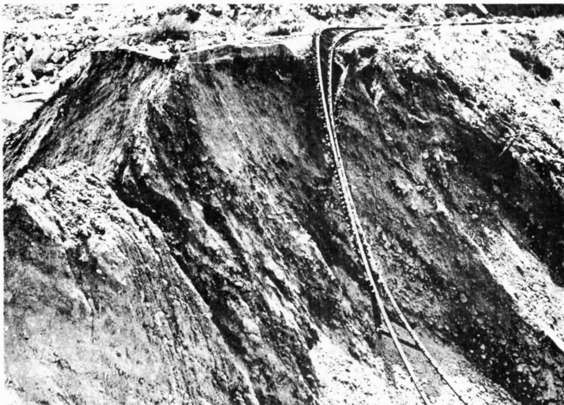
Three trestles were washed out and five others damaged during the storm, leaving trackage dangling in some areas on the rugged back country line.
