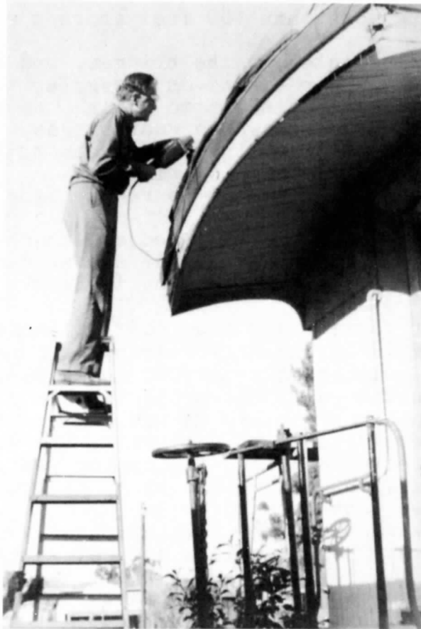
Dick McIntyre removes over 80 years of grime from the roof of D & R coach #14 at Poway.(L.Rose)
